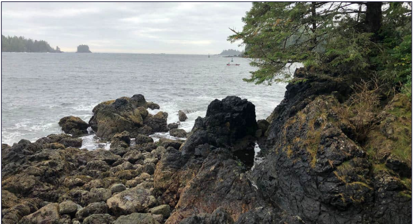
Figure 2.8.2 – Typical Foreshore Conditions (Southeast Side, View Looking South)
