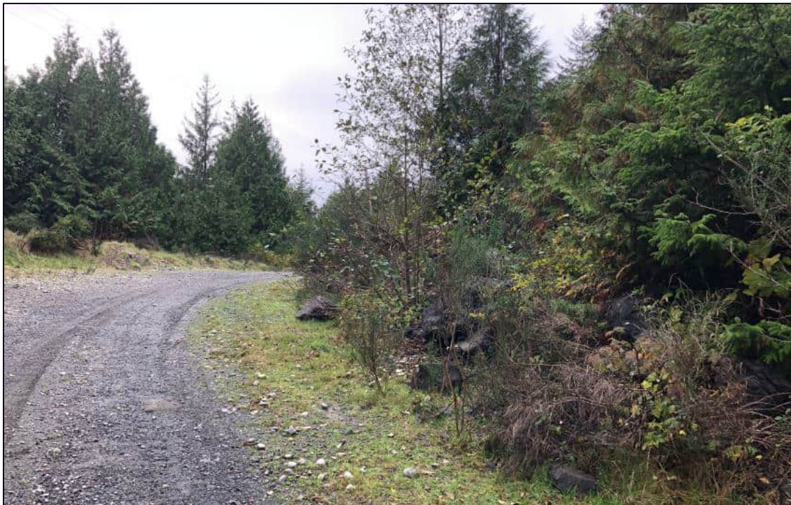
Figure 2.2.1 – Typical Terrain Conditions – Helen Road Extension (View Looking North)
